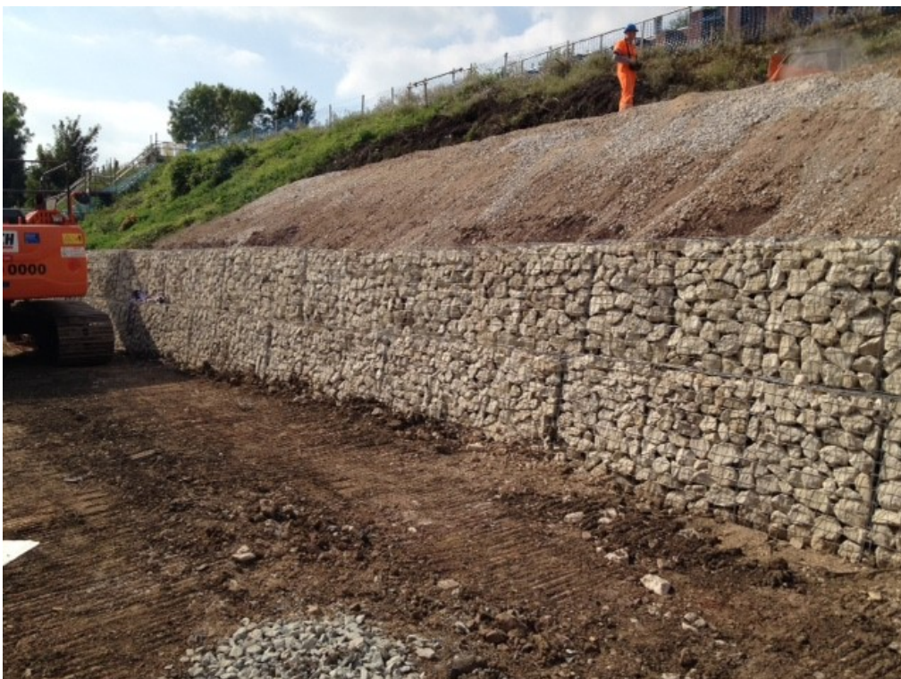
Figure 3: Gabions as secondary retention system
