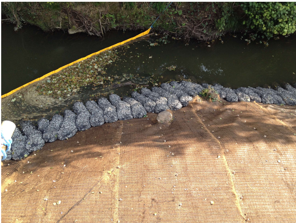
Figure 2: Rock rolls in conjunction with coir matting
