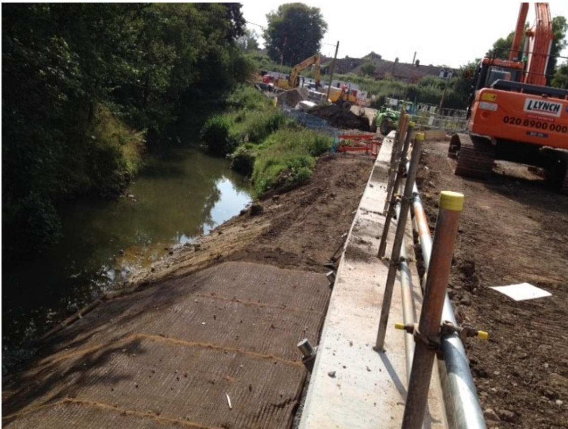
Figure 1: Coir matting to adjacent River Yeo bank
